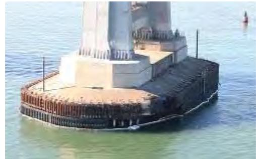
The Cosco Busan collision destroyed the bumper on one of the towers of the Bay Bridge. The new bumper cost Caltrans \$1.5 million to fix.
