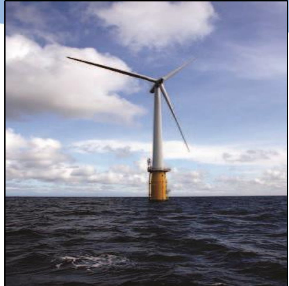
Statoil – 2.3 MW Turbine Deployment in Norway - 2009 Hywind-I Spar Substructure
