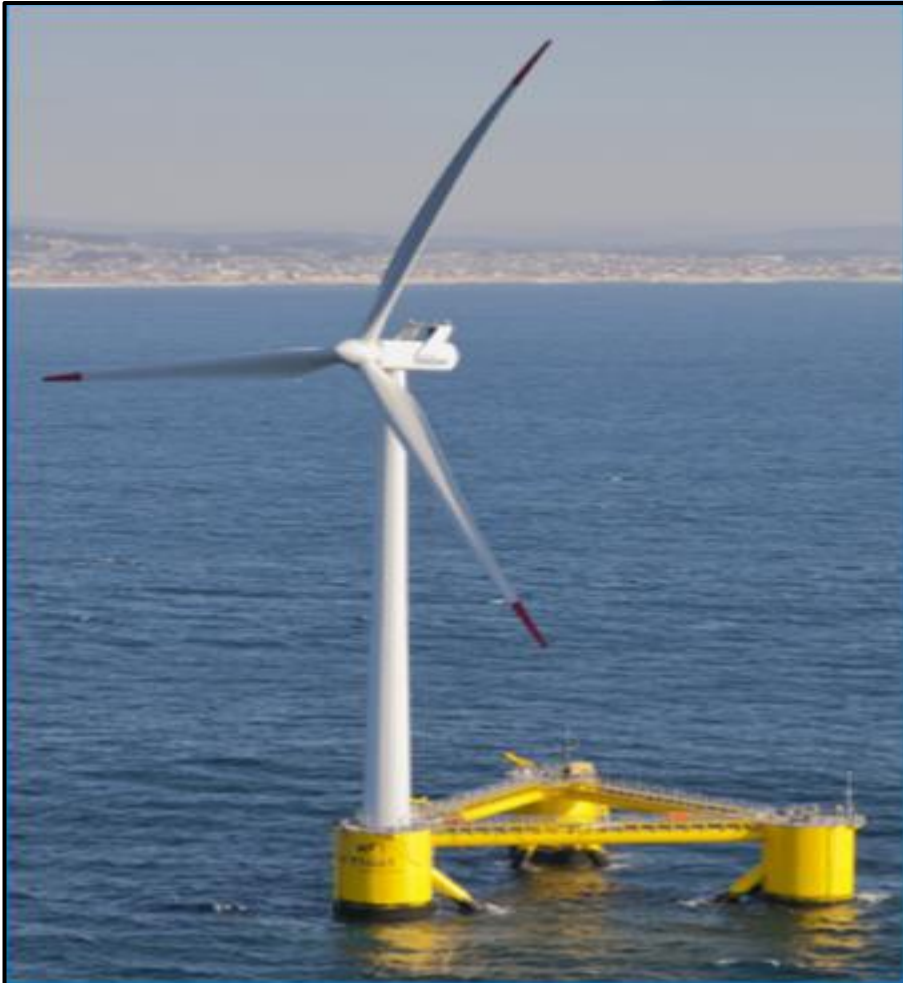
Principle Power – 2.0 MW Turbine Deployment in Portugal - 2011 WindFloat Semisubmersible Substructure
